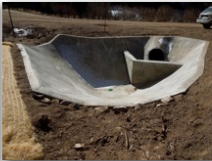
Sediment Catchment Basin
